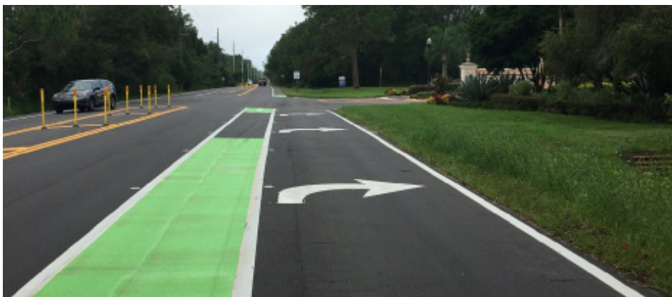
Cory Lake Boulevard was resurfaced, and the right of way was used to create a right-turn lane to reduce rear-end collisions and congestion.
