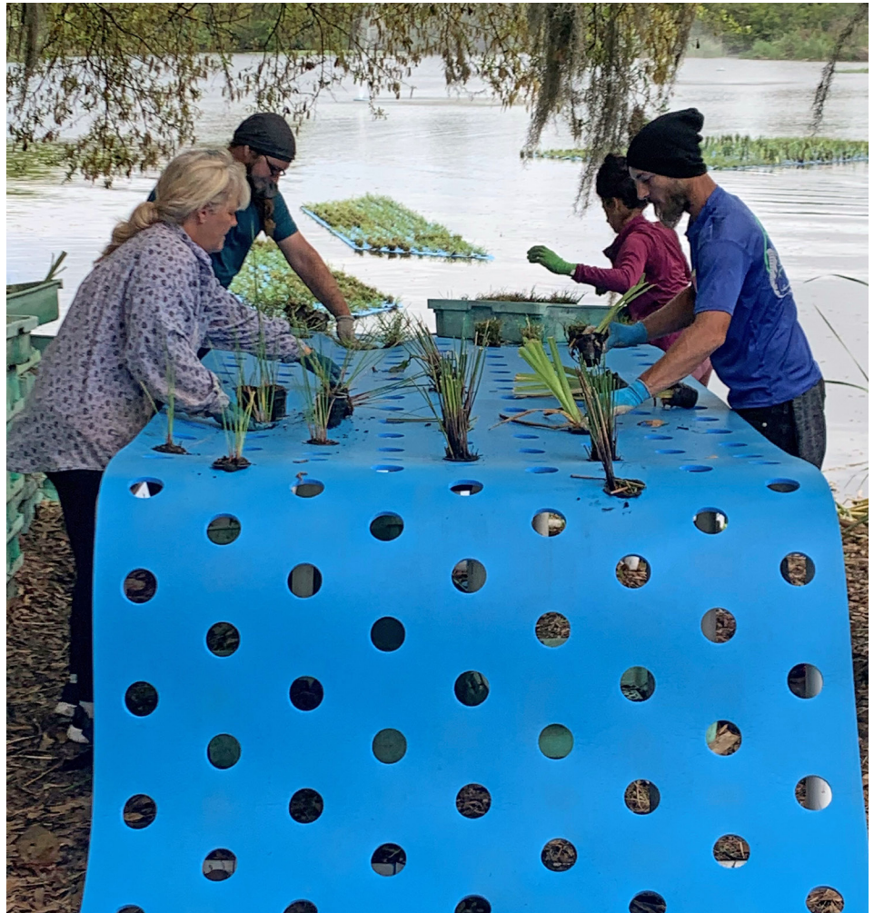
A floating wetland treatment system is installed in a South County stormwater pond.
