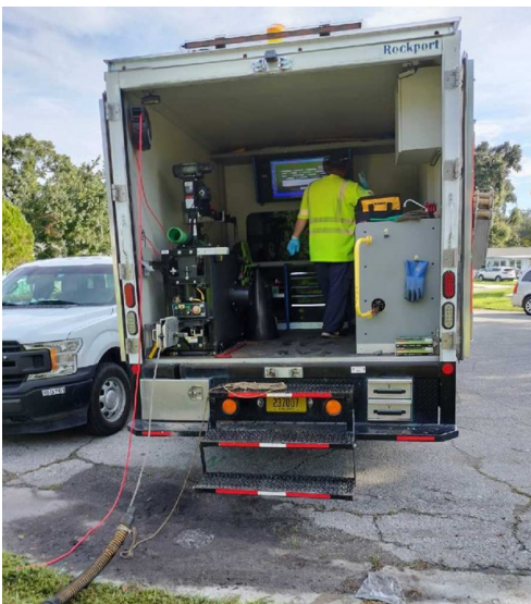
Field Operations conducts FELL inspections with electro scan equipment.
