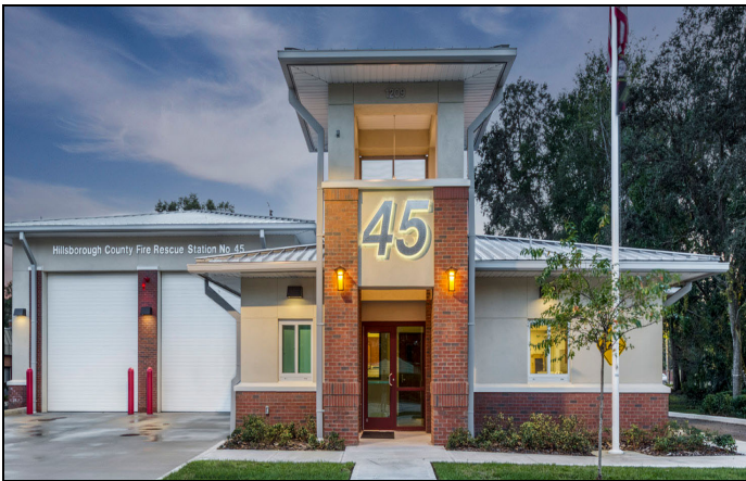
Central Brandon Fire Station #45
