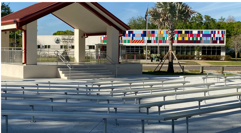
A new amphitheater and gazebo at Veterans Memorial Park provide a wonderful venue for outdoor events.
