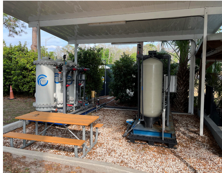
Far left: County staff work with electro scan equipment.
