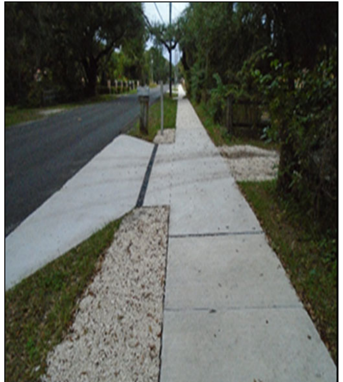
Sidewalk Repair Program
