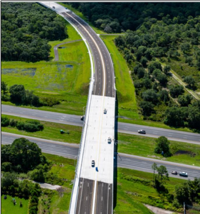
Apollo Beach Blvd I-75 Overpass
