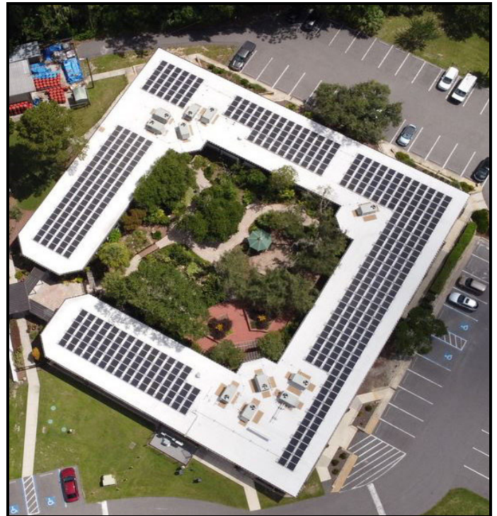
Solar Panels – Cooperative Extension Office
